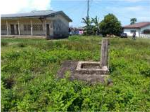
GNS Idenau School tap never flowing
